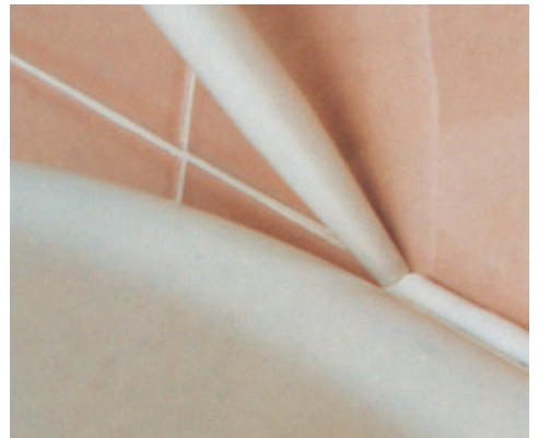
Sealing sanitary ware
