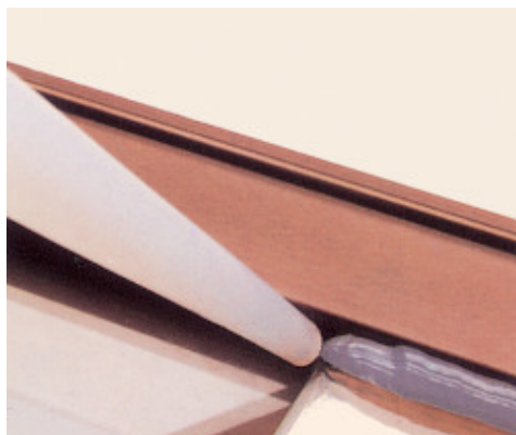
Sealing aluminium window frame with Mapesil AC-SC
