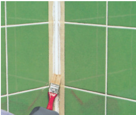
Smoothing the joint with Ultracare Smooth Silicone and a small brush
