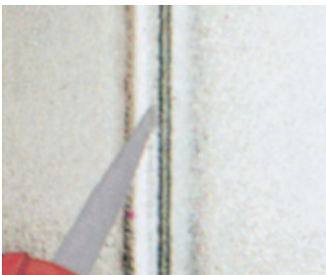
Sealing U-profile glass
