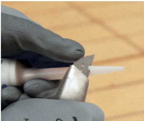
Cutting the nozzle according to the size of the joints
