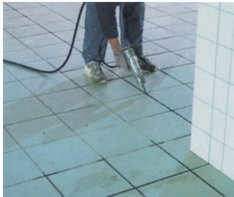
Sealing ceramic tile floor with Mapesil AC-SC
